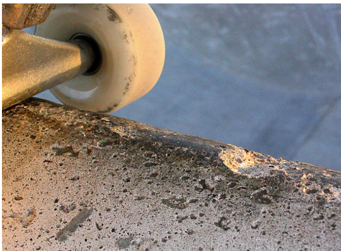
Chunked coping: Sumner, WA. The bike peg hit the coping as the rider was bailing a trick. Chunk fell to the bottom with the bike.
